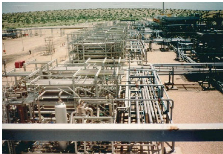
Figure 8.10 Photograph of the 500-million scfd CO 2 removal plant installed by UOP at Kandanwari, Pakistan. The UOP Separex system reduces CO 2 content of a natural-gas stream from 6.5 to 2% CO 2 . Photo used courtesy of UOP, LLC.
