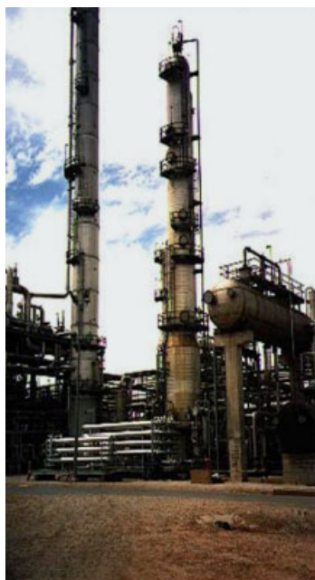
Figure 7.4 Air Liquide/Medal membrane unit replacement of amine scrubbing towers (used with permission).
