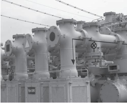
Figure 1. Gas-insulated switchgear (GIS).
